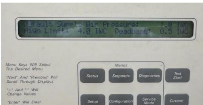
6. Setpoints of duct static pressure for a supply air fan
