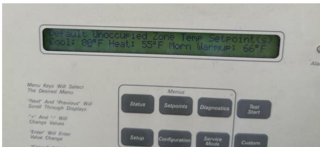
2. Optimized cooling and heating temperature setpoints for unoccupied hours of operation.
