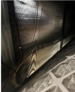
Tuneup (cleaning) of a HVAC unit's coils
