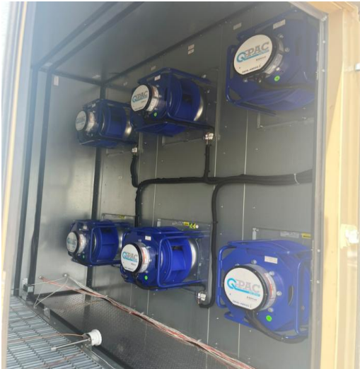
Electrically Commuted (EC) motor array
