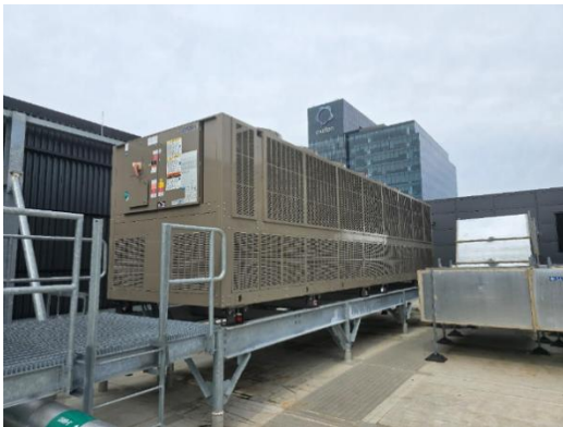
Air cooled chiller and outside air handling units
