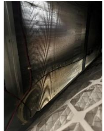
Tune-up (cleaning) of an HVAC unit's coils
