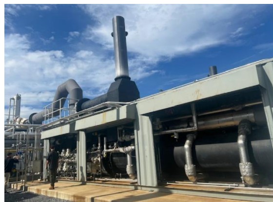
Heat Recovery Steam Generator
