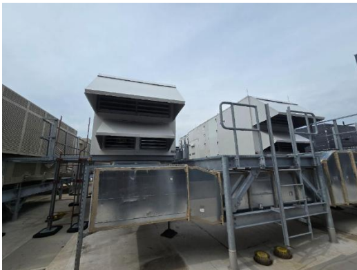
Air cooled chiller and outside air handling units
